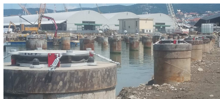
Figure 4. Double curved surface slider installed on site.
