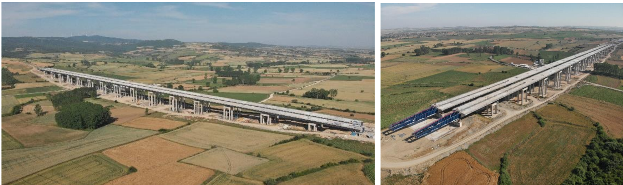
Fig. 7 - V06 viaduct under construction
